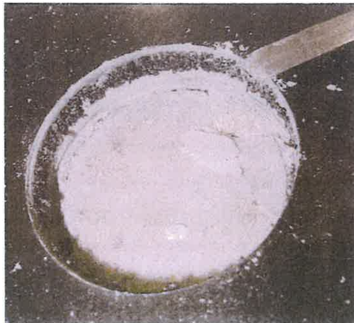
Figure 4. SignaFlor core #1 cavity. Part of the moisture mitigation membrane firmly attached to concrete.
