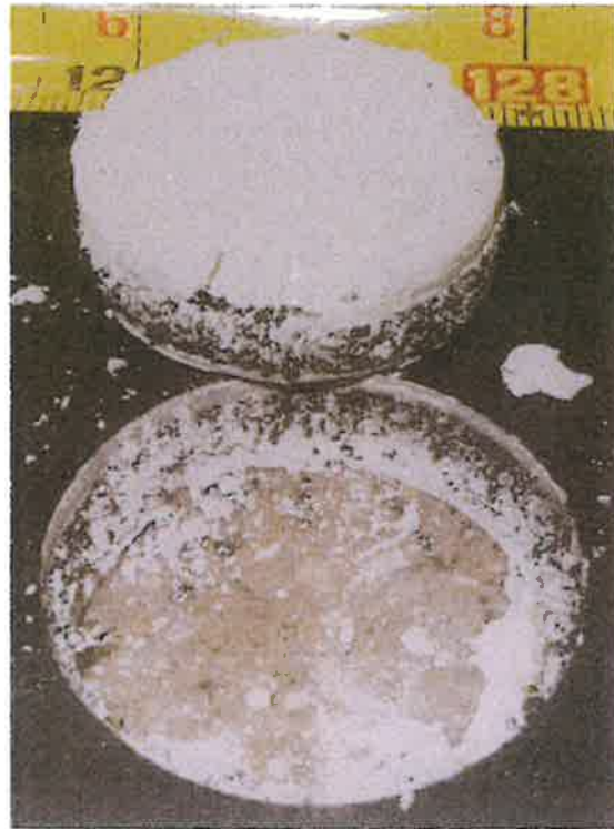
Figure 3. SignaFlor core #1 showing inverted core and cavity after removal.
