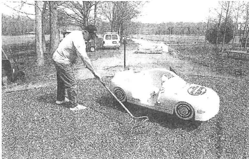
Raking loose-fill engineered wood fiber material
